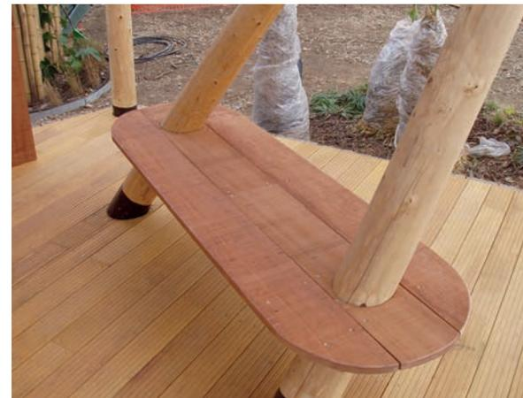
***Clockwise from top left: planed round timber bi-pod mast and tie pole (suitable for a pre-school) with cotton membrane; aged planed round timber with stainless guy and PVC membrane; planed round timber tripod with bench seat; planed round timber pole with galvanised bracketry and guy with natural cotton membrane; debarked pole with stainless bracketry and guys with natural cotton membrane***
